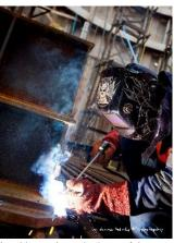
A welder works at the base of the South Tower before a concrete pour.
