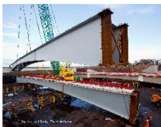
Girders are craned into position.
